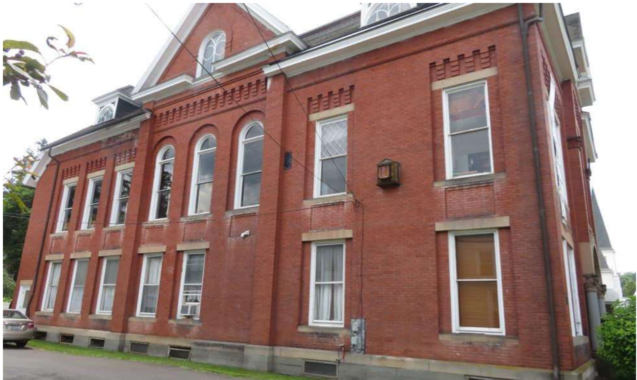
East façade as seen from Main Street
