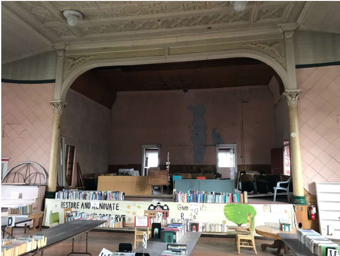
Second floor Opera House proposed for future renovation/restoration
