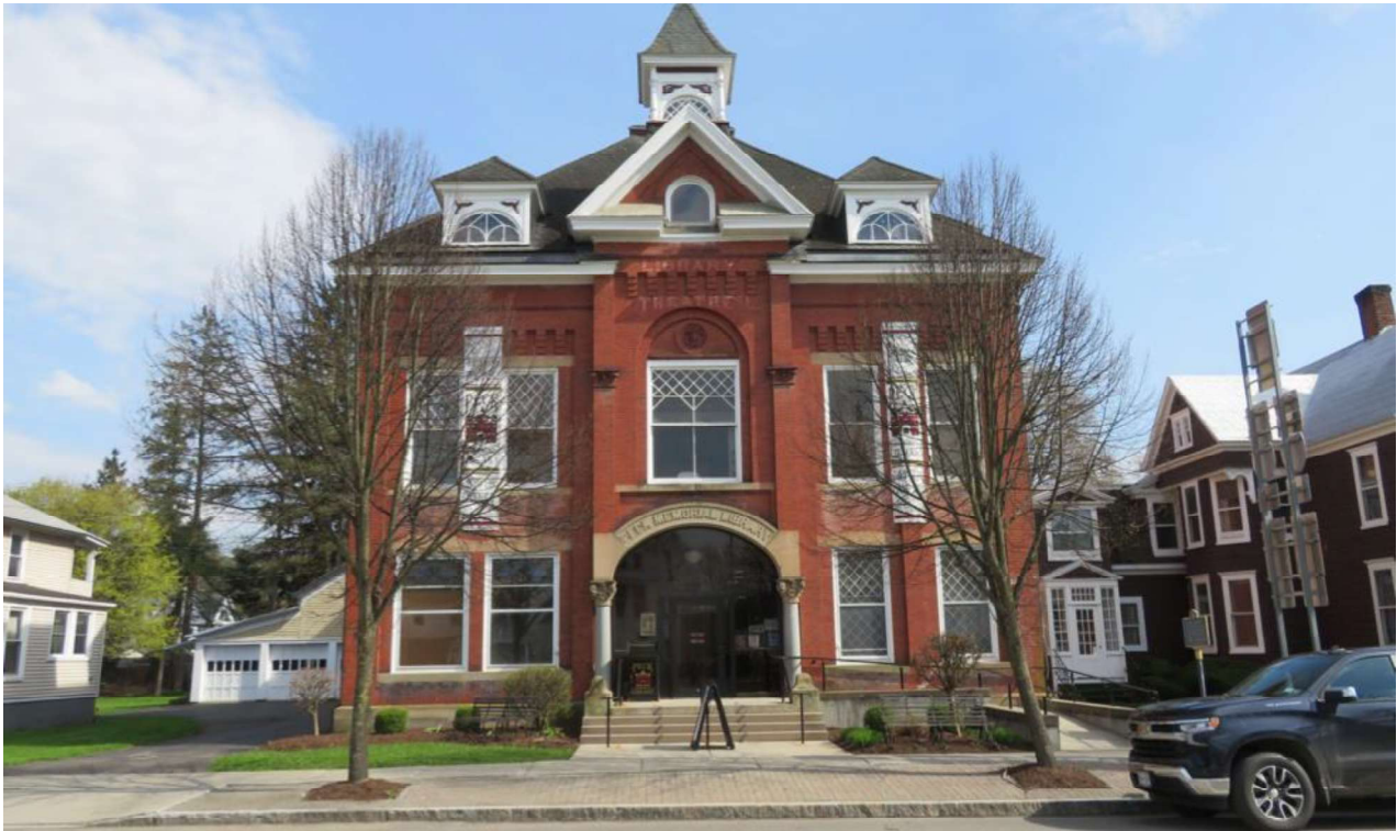
Front (north) façade as seen from Main Street (Spring 2025)
